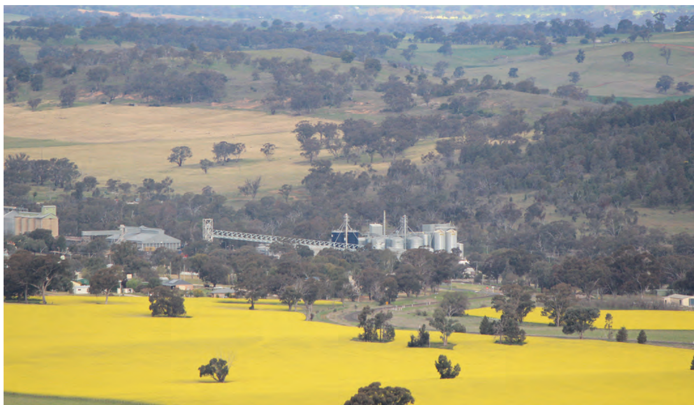
Image: MSM Milling's canola processing facility in Manildra, NSW.
