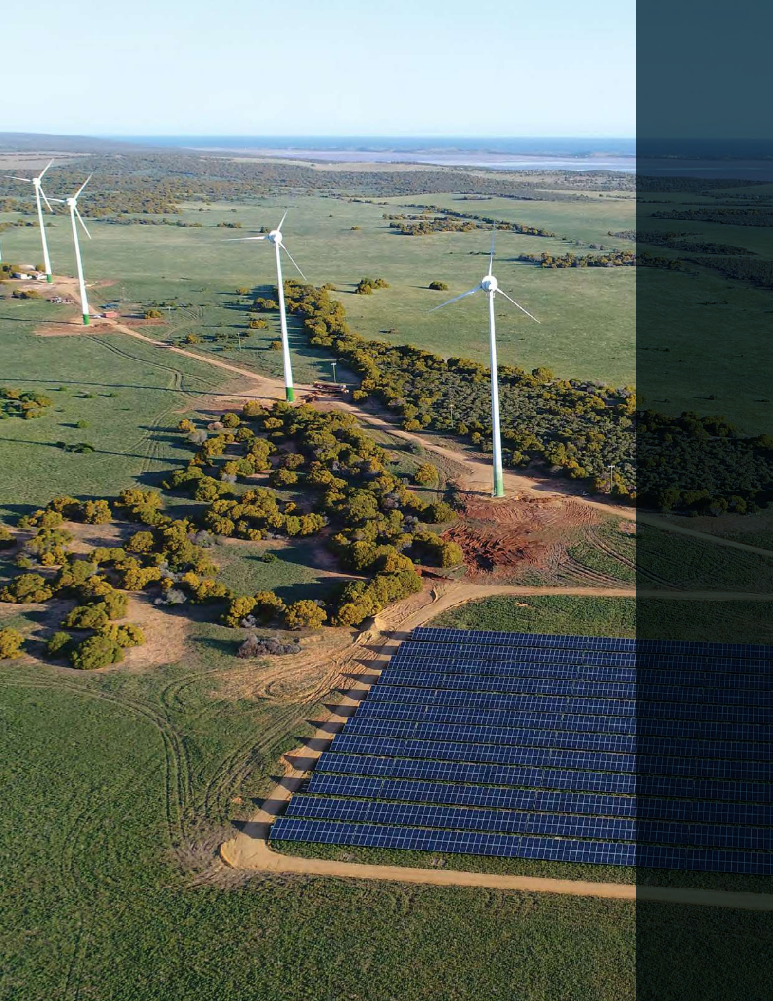
Advanced Energy Resources' 3.5 MW wind and solar farm with battery storage at Port Gregory in Western Australia. Image credit: Advanced Energy Resources.
