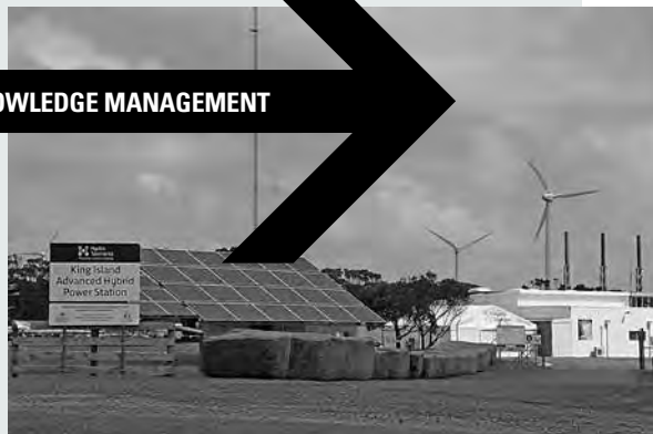
The King Island Advanced Hybrid Power Station
